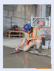
art of applying various finishes to concrete surfaces such as architectural, exposed, acidstained, patterned, broomed finish overlays, and smooth finishes. Trainees will be taught to use hand and power tools such as floats and screeds.
